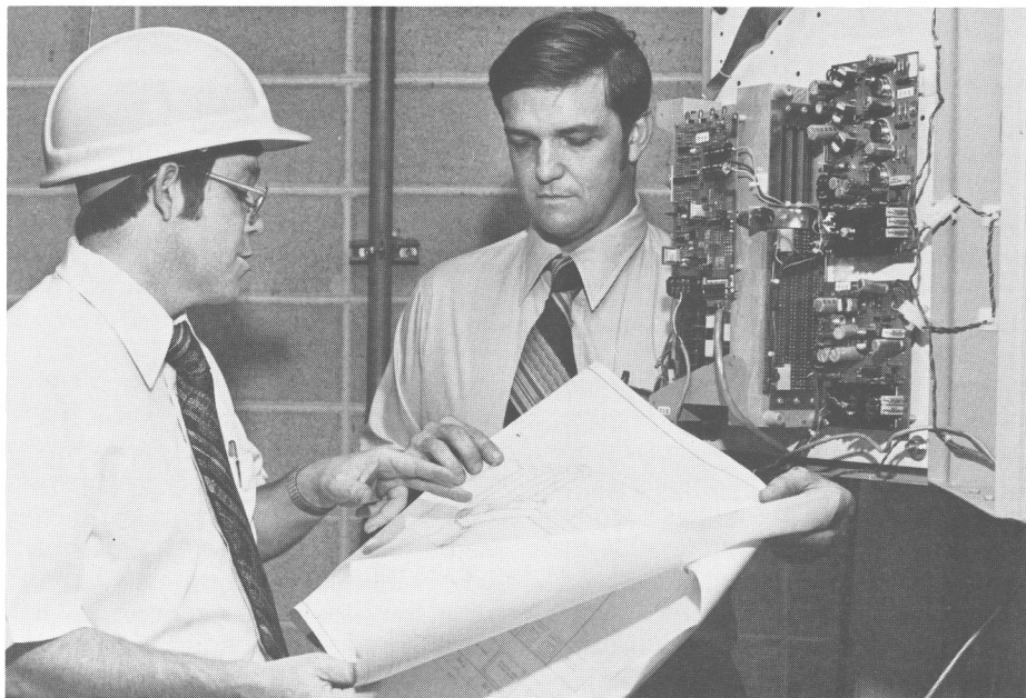
Don Alexander, Physical Plant, and John Scoville, ECSL, inspect part of the Facilities Management System they helped develop to reduce energy consumption on the Georgia Tech campus.
