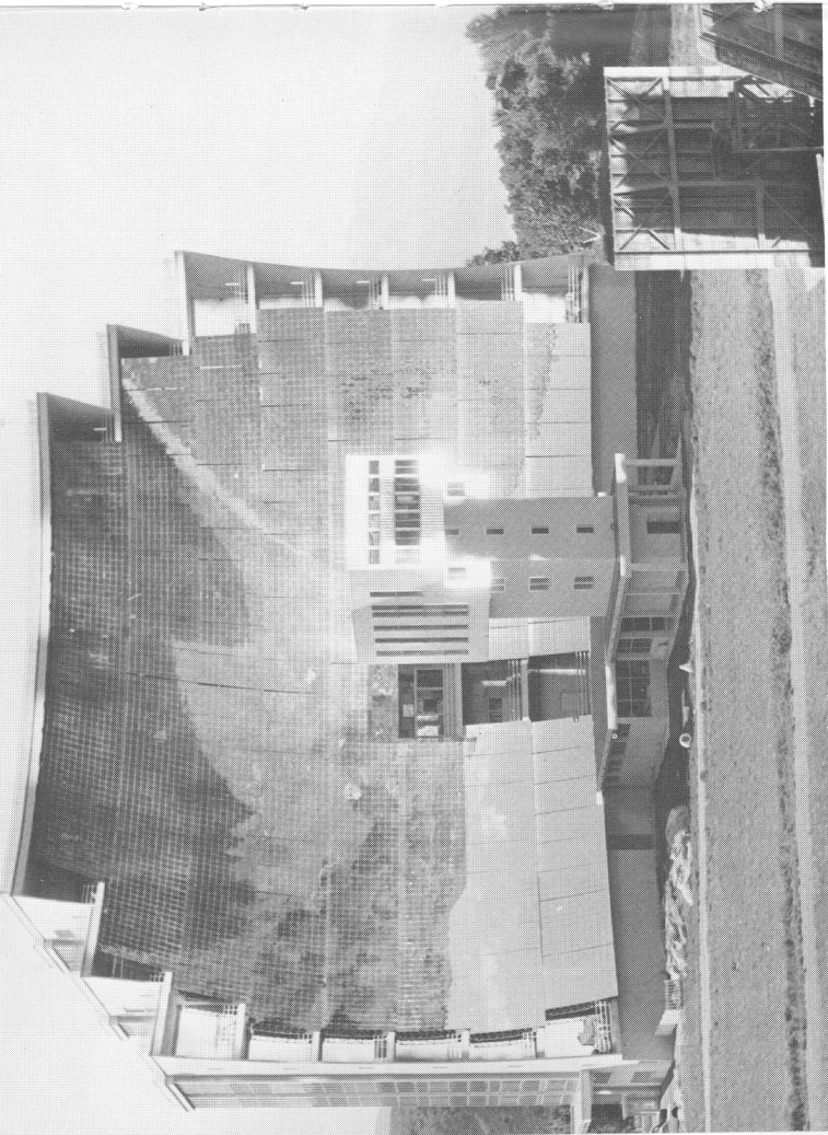
The CNRS Solar Furnace in Odeillo-Font Romeu, France, produces heat fluxes up to 7000° F.
