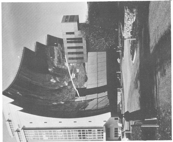
The CNRS Solar Furnace in Odeillo-Font Romeu, France, produces heat fluxes up to 7000° F.
