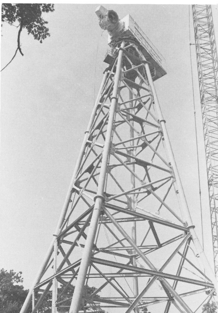
The Eiffel Tower? No, the NASA windmill tower, earmarked for EES radar research use. Anita Edwards of S&TL took this photo during dismantling, after removal of windmill blades.
