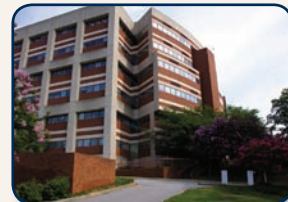
1985 – Coinciding with Georgia Tech's 100th birthday, GTRI moves into a new home, the $12.5 million, six-story Centennial Research Building.
