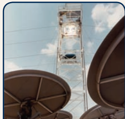
1977 – Solar energy research heats up at EES with construction of a 325-kW, 500-mirror Solar Thermal Test Facility, the second largest in the U.S.
